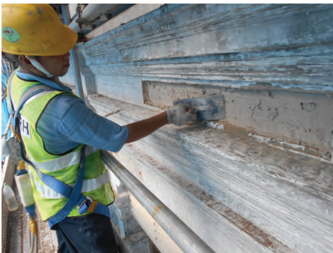
Mapei-Antique MC was applied for built-up thickness.
