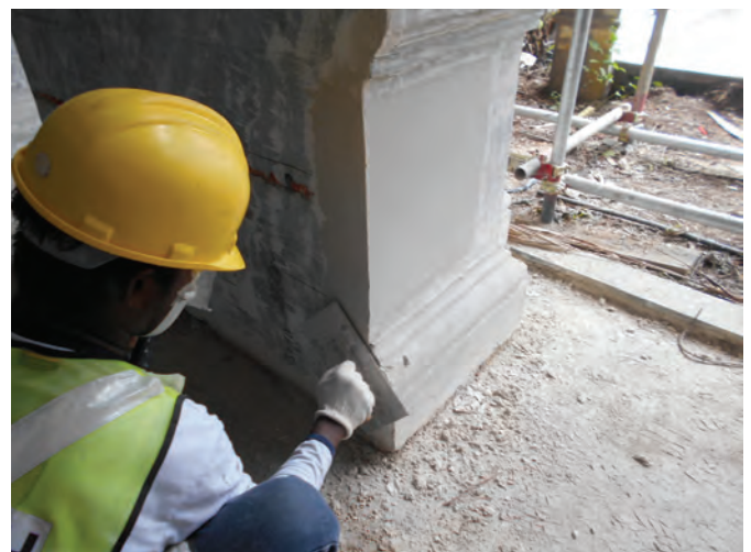
Mapei-Antique FC was applied to give a smooth finishing.
