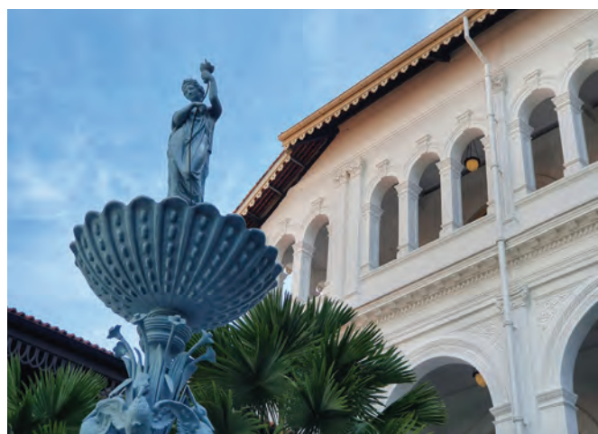
TOP AND ABOVE: The latest restoration work aimed to infuse technology for modern conveniences and update the interior while ensuring the hotel's unique historic charm would be preserved.
