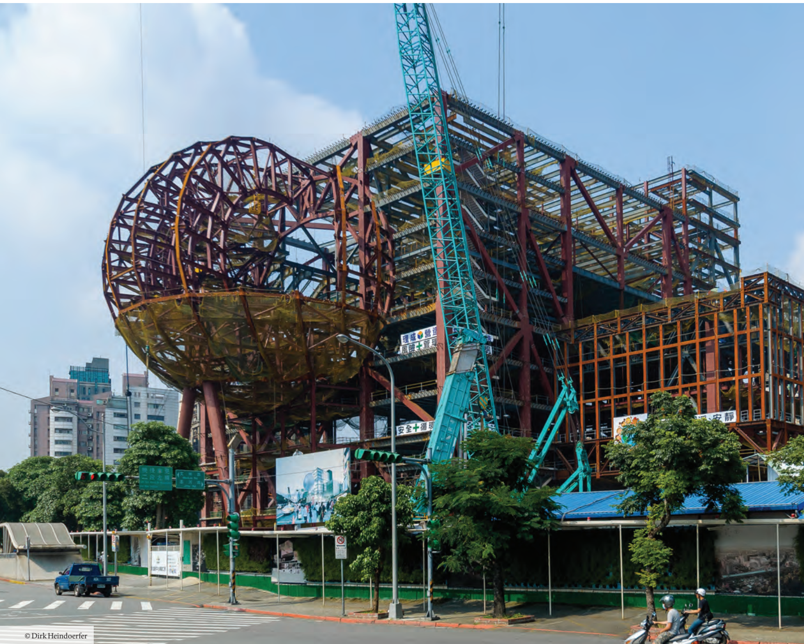
In the ellipsoidal Globe Playhouse, the 26-m cantilevering volume is framed by a three-dimensional space truss.
