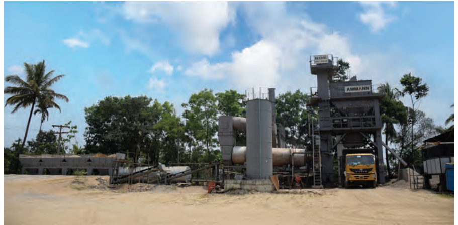
ABOVE AND BOTTOM: An Ammann ABC 120 EcoTec asphalt plant is designed for ease of operation and maintenance. NDE Readymix uses the standard plant configuration, which has served the company well.
